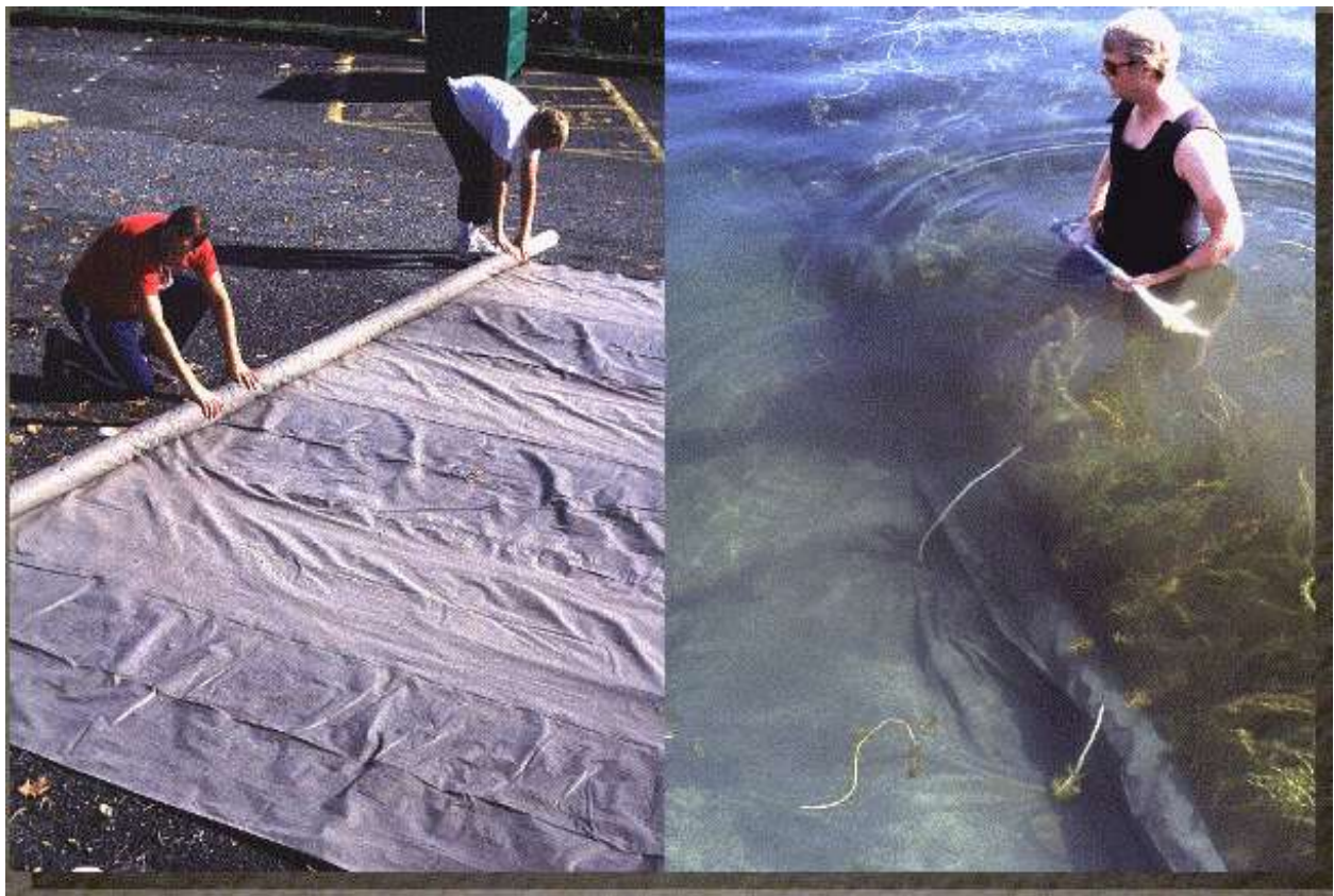
Benthic barriers being installed on an inland lake.
