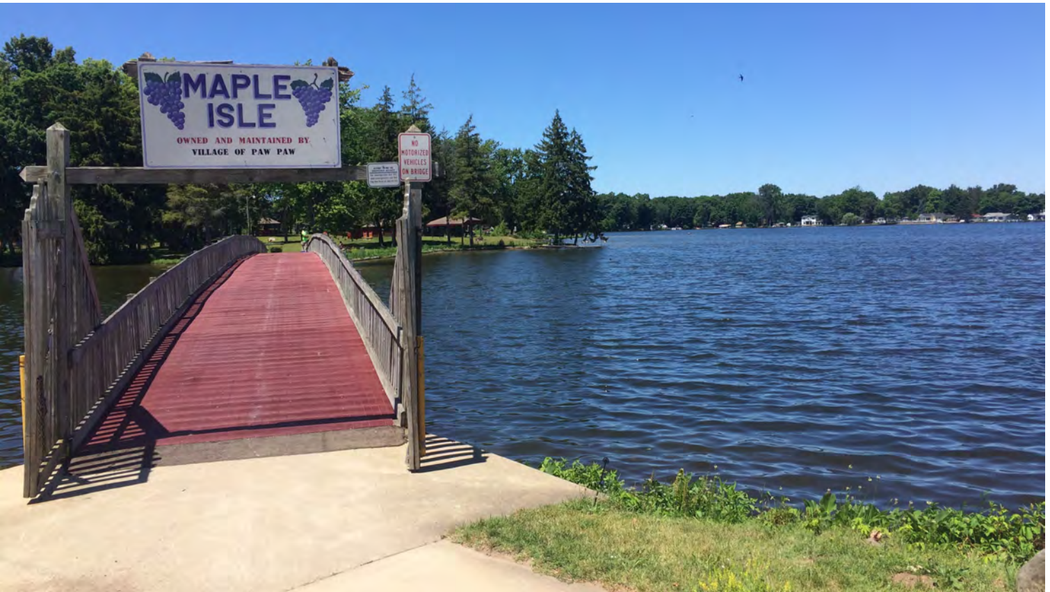
Pedestrian bridge to Maple Island over Maple Lake
